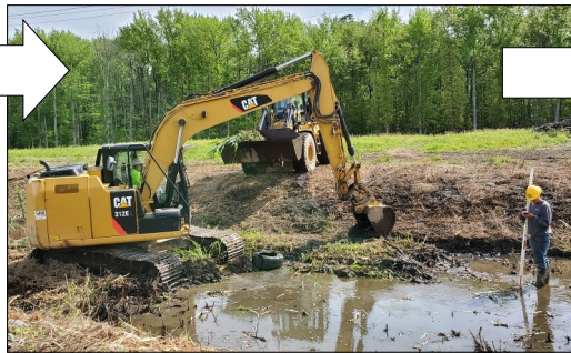
Sediment being removed from ditch
