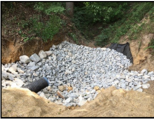
Gully erosion repaired
