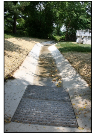
Concrete gutter replacement behind homes in School Bell Gardens
