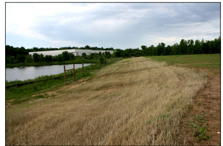
Erosion control work in 2018
