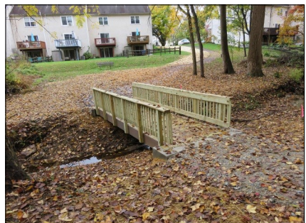
Pedestrian trail and footbridge in the community of Richards Lane
