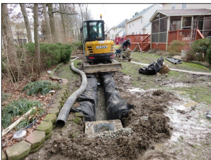
Backyard drainage system installed in Timber Farms
