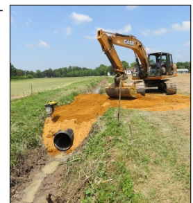
Pipe installation on Massey’s Tax Ditch
