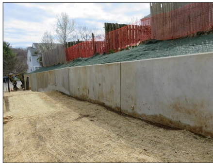
Concrete retaining wall replaced old timber wall in Drummond Ridge
