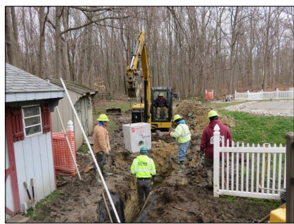
Drainage system installed in soggy area behind homes in The Oaks
