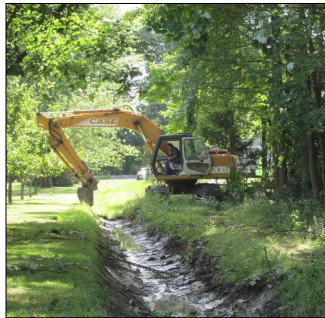
Jeff working on Guthrie Tax Ditch maintenance mowing and ditch clean-out
