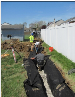
Backyard drainage system installed in Rutledge
