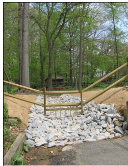
Rock-lined swale installed at home in Chalfonte
