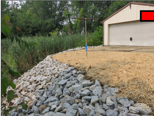
Drainage inlet installed and embankment stabilized for landowner adjacent to marsh land in New Castle.
