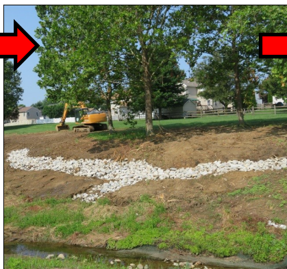
An embankment behind homes in Colton Meadows backing up to the stormwater pond was cleared of vegetation and some spots stabilized with riprap to enable the HOA to begin regular maintenance to maintain visual views to the pond.
