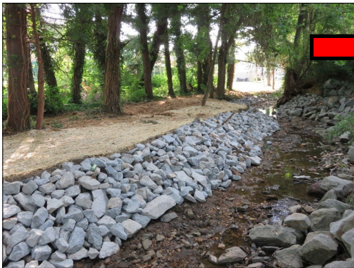
An eroding urban channel in the development of Maplecrest was cleared of vegetation, re-graded and stabilized with riprap.
