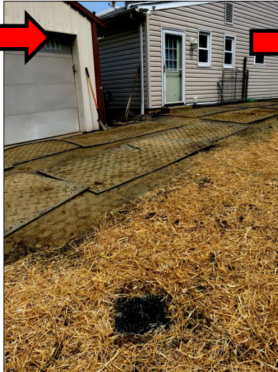
Drainage inlet installed and embankment stabilized for landowner adjacent to marsh land in New Castle.
