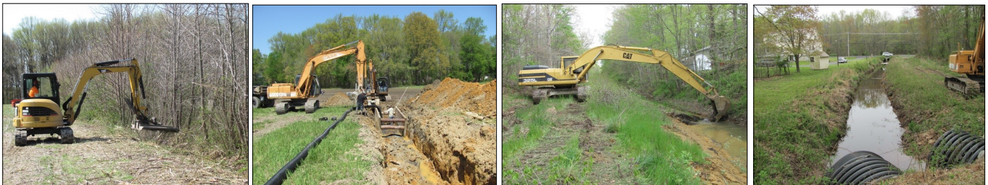
From L to R: mowing vegetation on Brennan-Berry Tax Ditch, tile line replacement on Sandom Branch Tax Ditch, dipping out sediment in the Woods Road Tax Ditch, and ditch cleanout on the main stem of the Pencader Tax Ditch.
