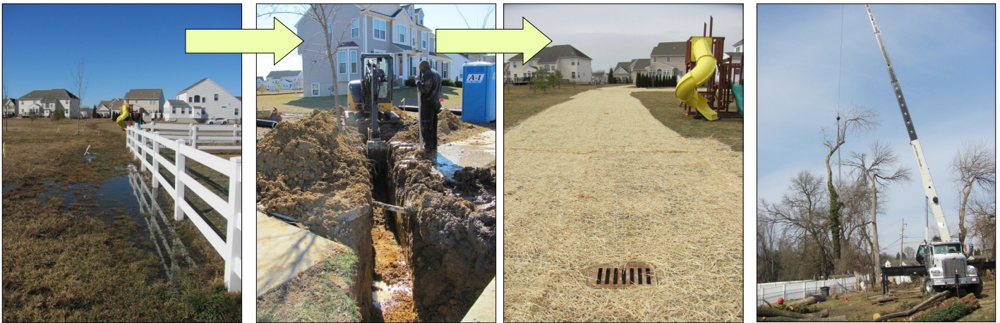
From L to R: wet soils behind homes in Odessa National remediated with the installation of a pipe and catch basin drainage system. Tree removal in rights of way behind homes on Newport Gap Pike near Brandywine Springs Park. Future drainage work is planned.
