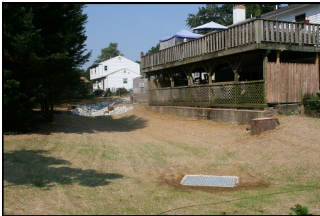
Drainage channel partially piped and upper end protected with stone for landowner in Piermont Woods near Newark
