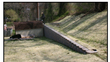
Wall installed to stabilize slope
