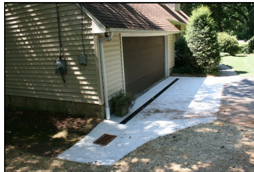
Slotted trench drain in driveway of a property in Crestfield, North Wilmington
