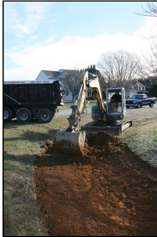
Re-grading an existing swale in Summit Bridge Farms
