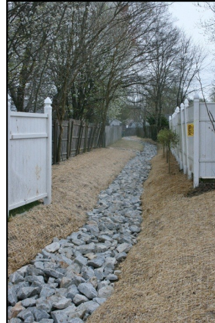
Existing drainage easement cleaned out and lined with riprap in Breezewood II
